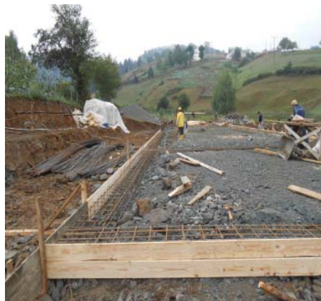
Foundation Formwork, Concrete Steel and Concrete Works
